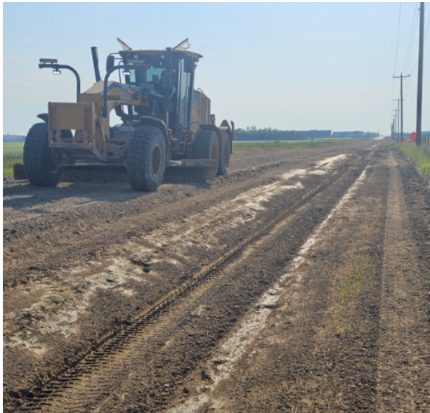
Before: Shoulder pull and soft spot repair at Township Road 500 between Range Road 245 and Range Road 250
