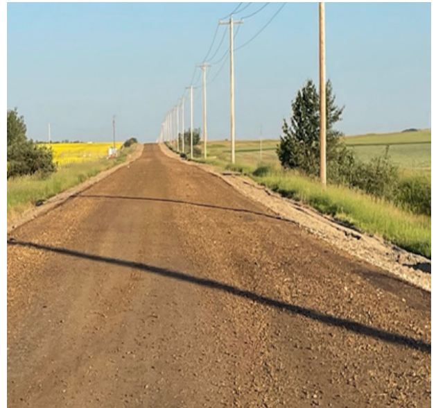
After: Shoulder pull and soft spot repair at Township Road 500 between Range Road 245 and Range Road 250
