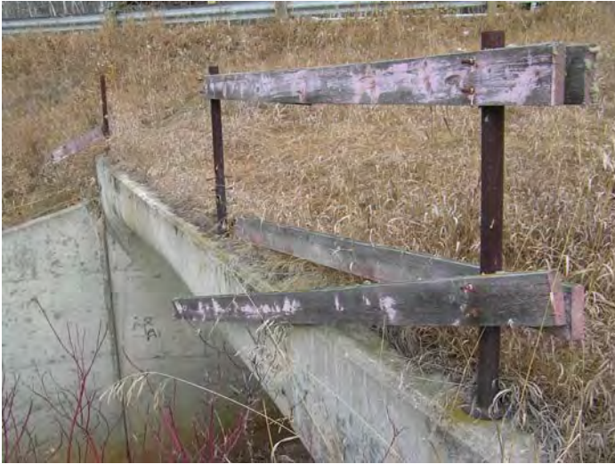
Broken rail at top of inlet
