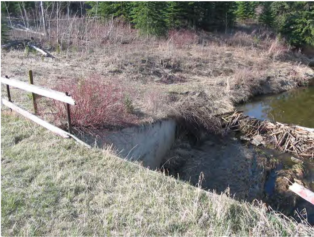
Inlet side (south) – barrier is broken.
