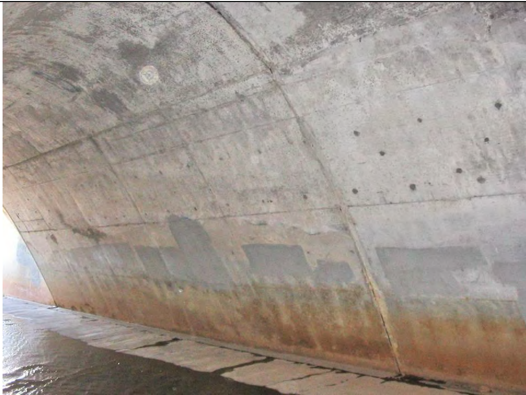
Interior wall of culvert. Minor cracking in base slab.
