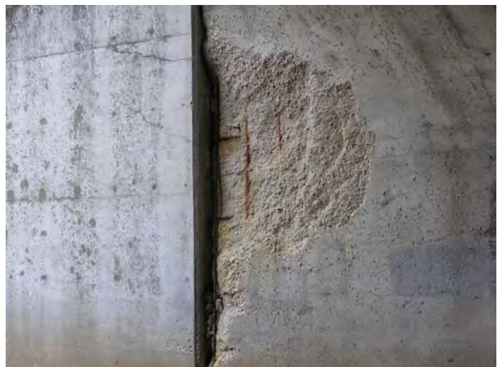
Large delamination area at NE end of barrel
