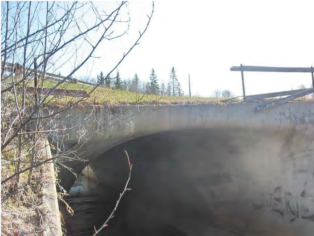
Upstream side of culvert showing broken barrier.
