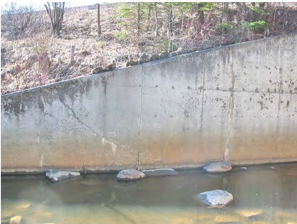
Wingwall with some cracking. Some staining but no evidence of corrosion.
