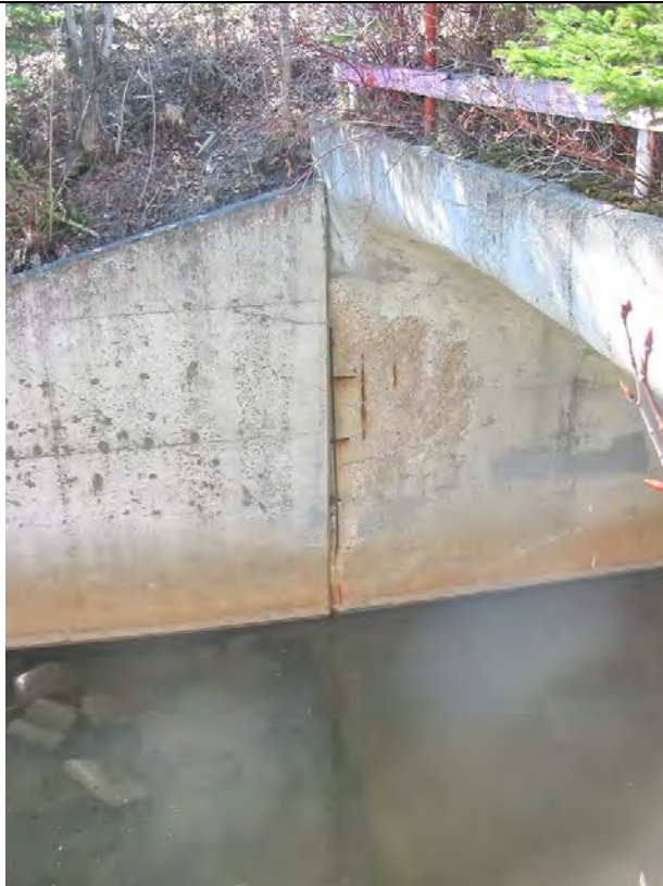
Concrete spall and exposed reinforcing steel – outlet of culvert.
