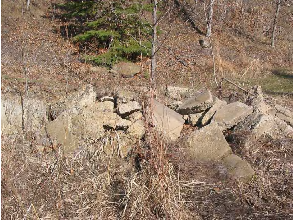
Concrete apron slab broken and used as rip rap
