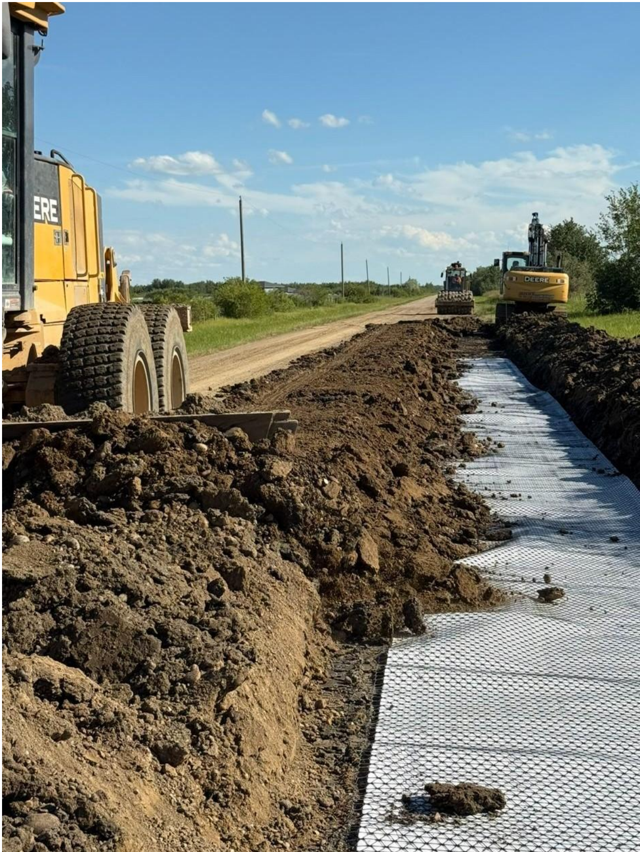
Soft shoulder stabilization with geogrid, Range Road 230
