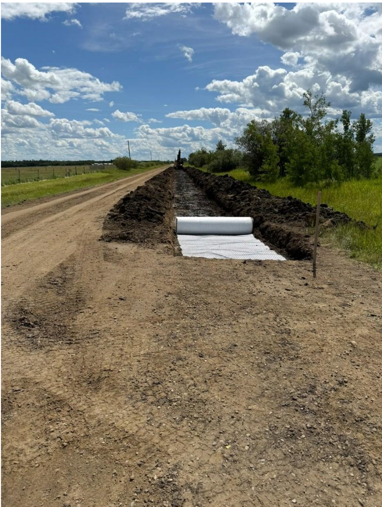
Soft shoulder stabilization with geogrid, Range Road 230
